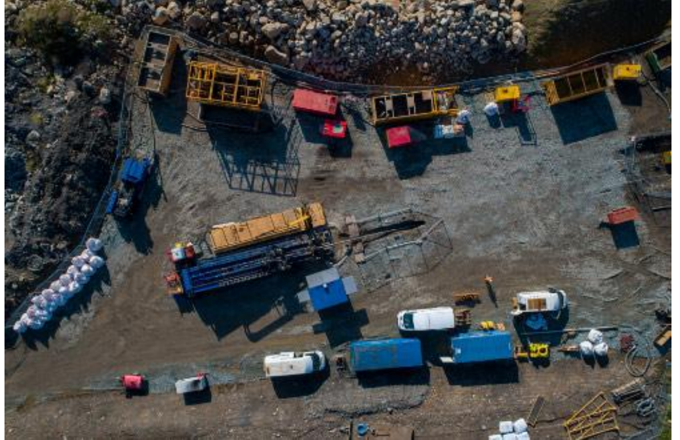
Typical HDD compound set up
