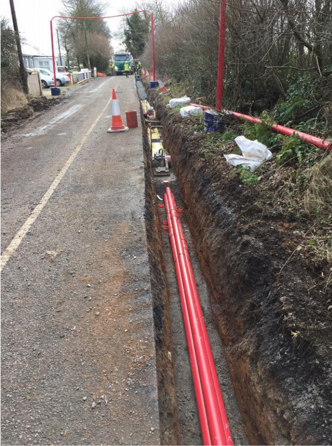
Typical underground cable installation
